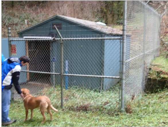
Photo 14: Pump and Disinfection Building
