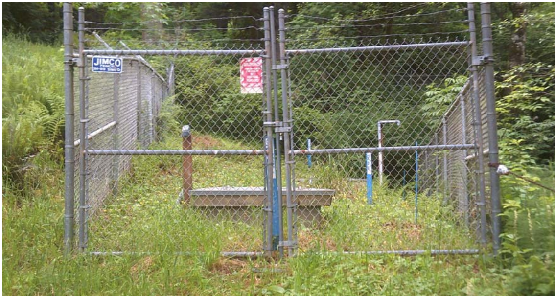
Figure 2- Spring 3 (Photo taken from south end of spring, looking north)
