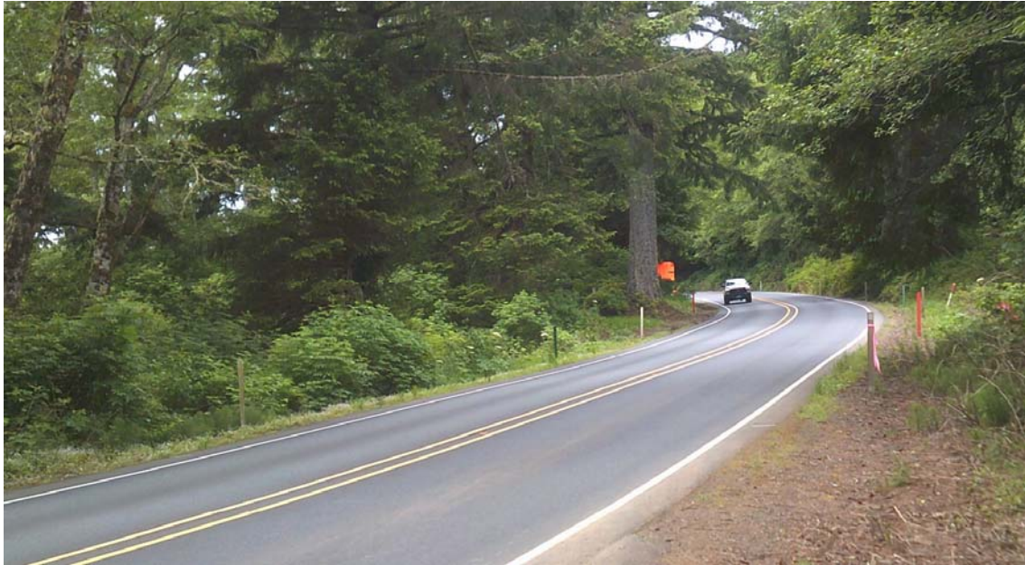
Figure 1 - Highway 101 above Spring 3 (Photo taken from east side looking north)
