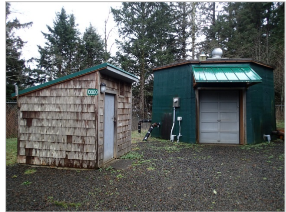
Photo 2: Treatment Building (right)
